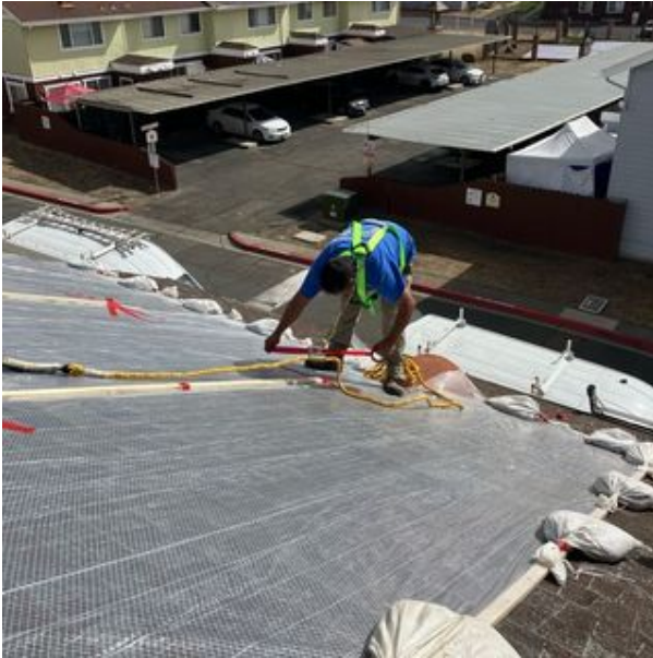
File Name:Roof tarp_0013.jpg Description:10-01-25 tarping roof HiRes Image URL: Click Me
