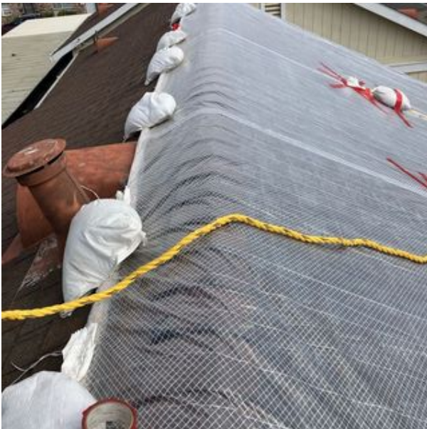
File Name:Roof tarp_0018.jpg Description:10-01-25 roof overview HiRes Image URL: Click Me
