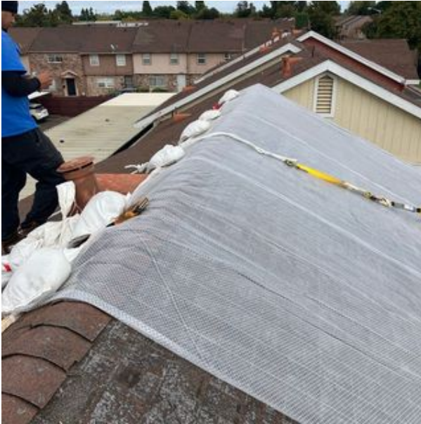
File Name:Roof tarp_0020.jpg Description:10-01-25 tarping roof HiRes Image URL: Click Me
