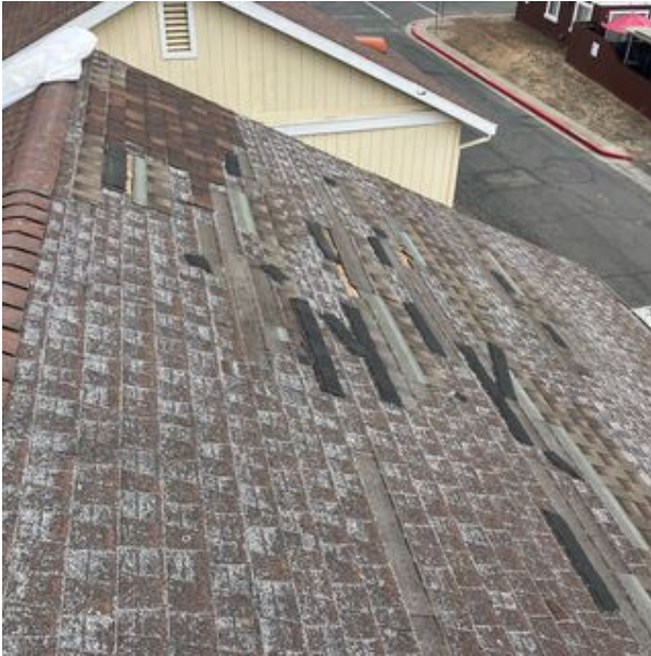
File Name:Roof tarp_0012.jpg Description:10-01-25 roof overview HiRes Image URL: Click Me
