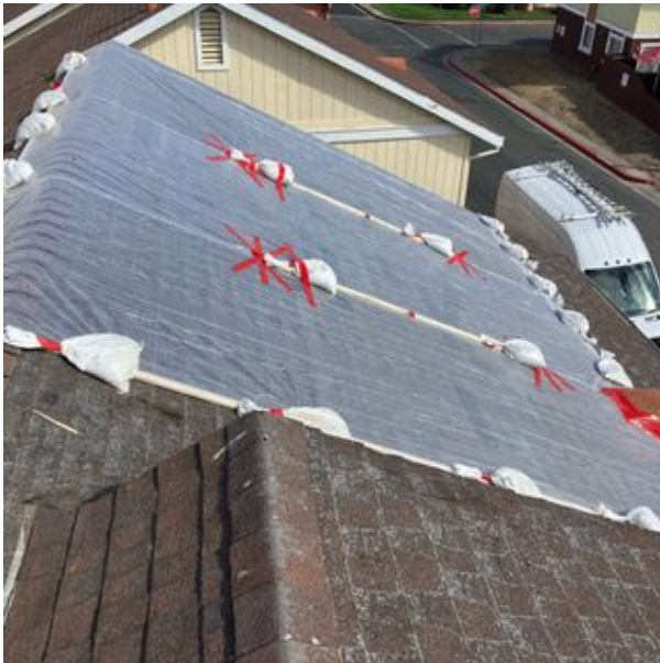
File Name:Roof tarp_0021.jpg Description:10-01-25 roof tarp HiRes Image URL: Click Me
