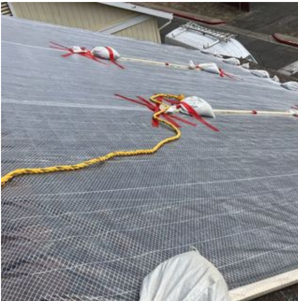
File Name:Roof tarp_0017.jpg Description:10-01-25 tarping roof HiRes Image URL: Click Me
