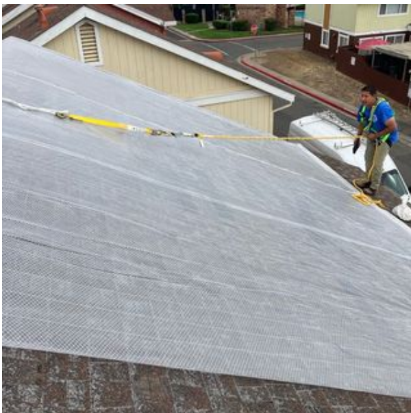
File Name:Roof tarp_0022.jpg Description:10-01-25 roof tarp HiRes Image URL: Click Me
