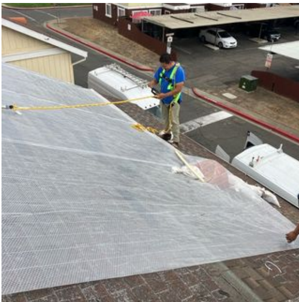
File Name:Roof tarp_0005.jpg Description:10-01-25 roof tarp HiRes Image URL: Click Me
