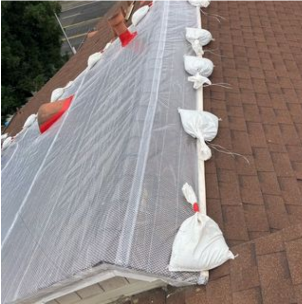
File Name:4149 tarp_0005.jpg Description:10-01-25. Unit 4149 Tarp roof HiRes Image URL: Click Me
