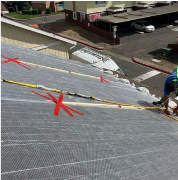
File Name:Roof tarp_0014.jpg Description:10-01-25 tarping roof HiRes Image URL: Click Me
