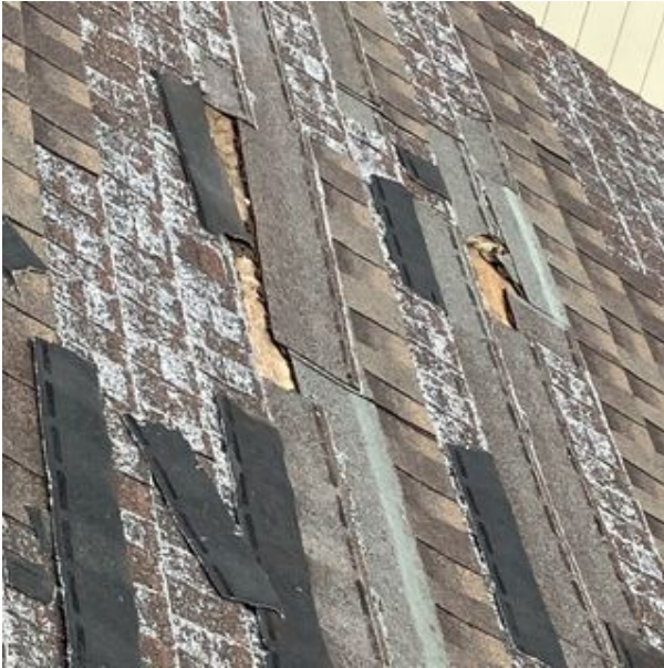
File Name:Roof tarp_0016.jpg Description:10-01-25 roof overview HiRes Image URL: Click Me
