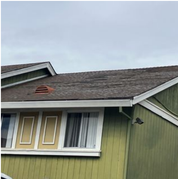
File Name:Roof tarp_0004.jpg Description:10-01-25 roof tarp HiRes Image URL: Click Me
