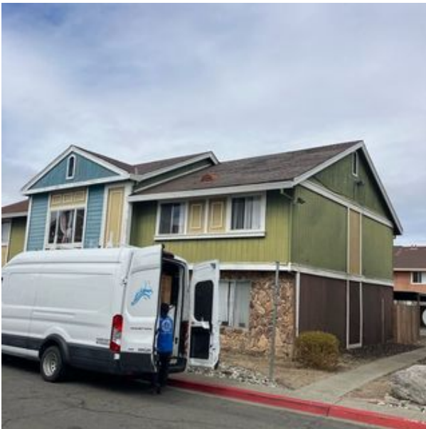
File Name:Roof tarp_0002.jpg Description:10-01-25 roof tarp HiRes Image URL: Click Me
