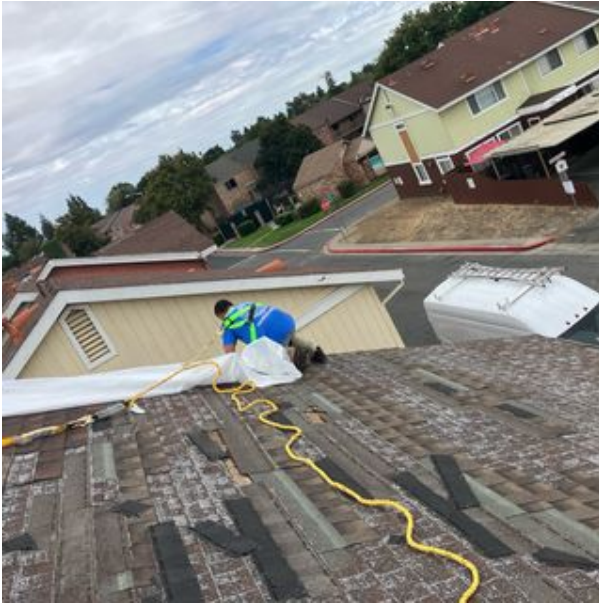
File Name:Roof tarp_0019.jpg Description:10-01-25 tarping roof HiRes Image URL: Click Me
