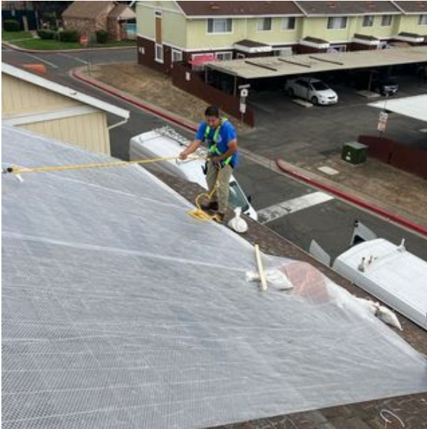
File Name:Roof tarp_0001.jpg Description:10-01-25 roof tarp HiRes Image URL: Click Me
